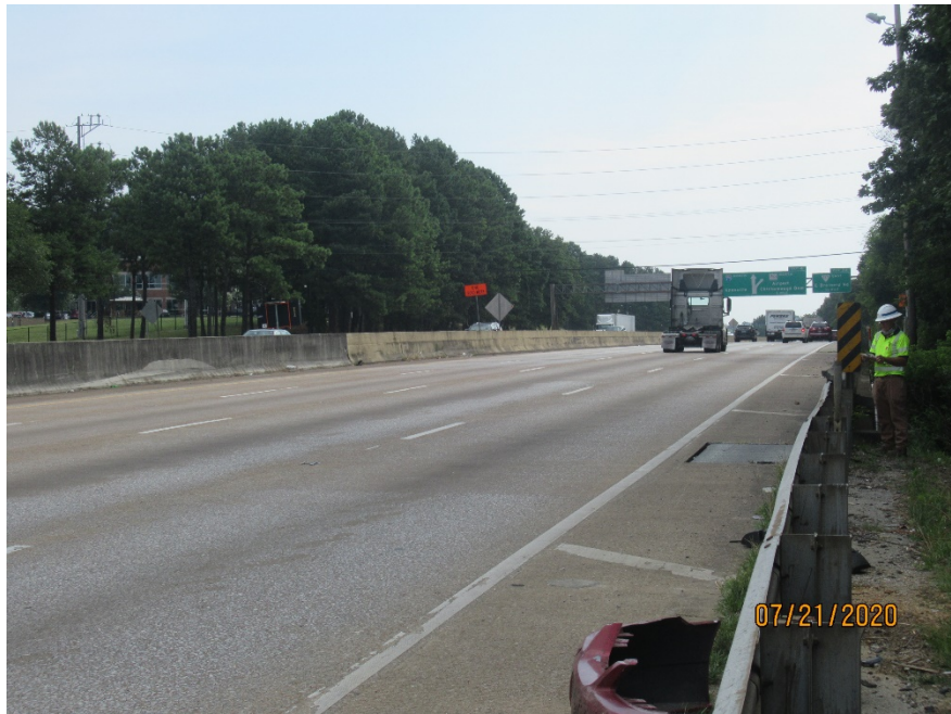
LOOKING AHEAD ON STRUCTURE - RT, NORTHBOUND
