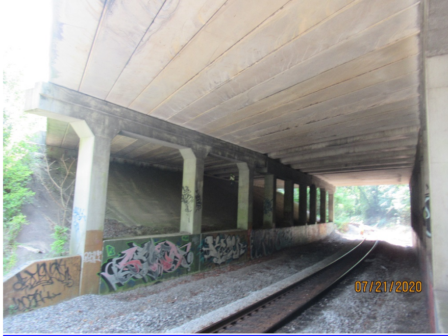
BOTTOM OF DECK
