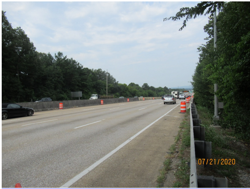
LOOKING BACK ON STRUCTURE - LT, SOUTHBOUND
