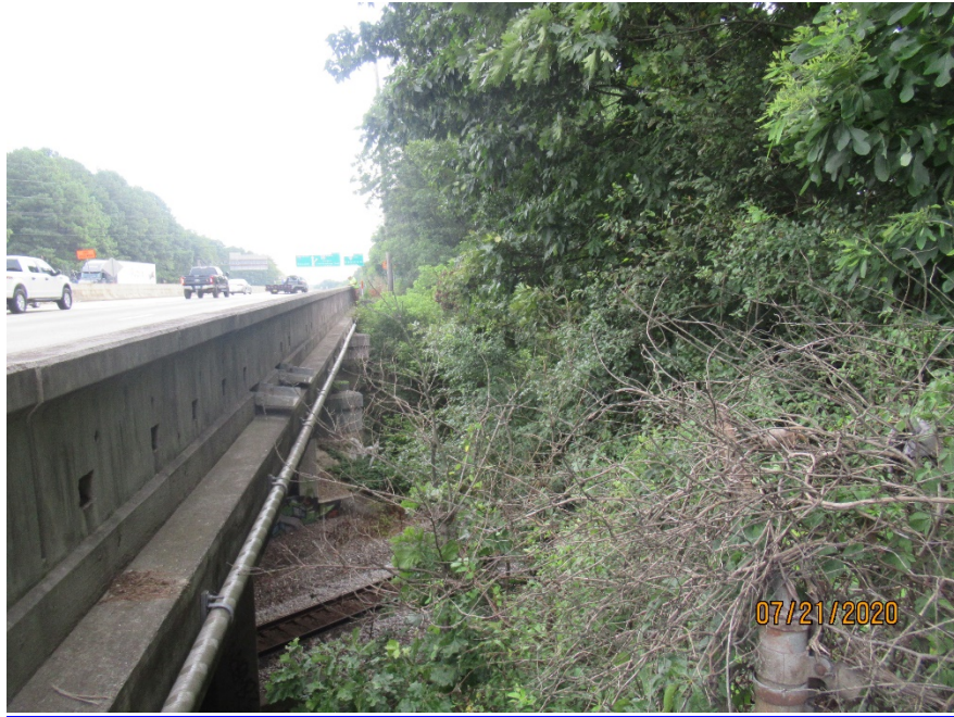
UTILITIES - BEAM "II" OVERHANG
