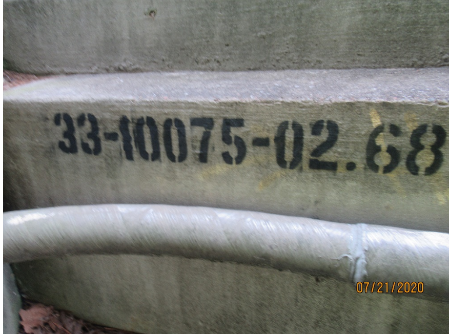
BRIDGE NUMBER - NUMBER 1, RT, BEAM "II"
