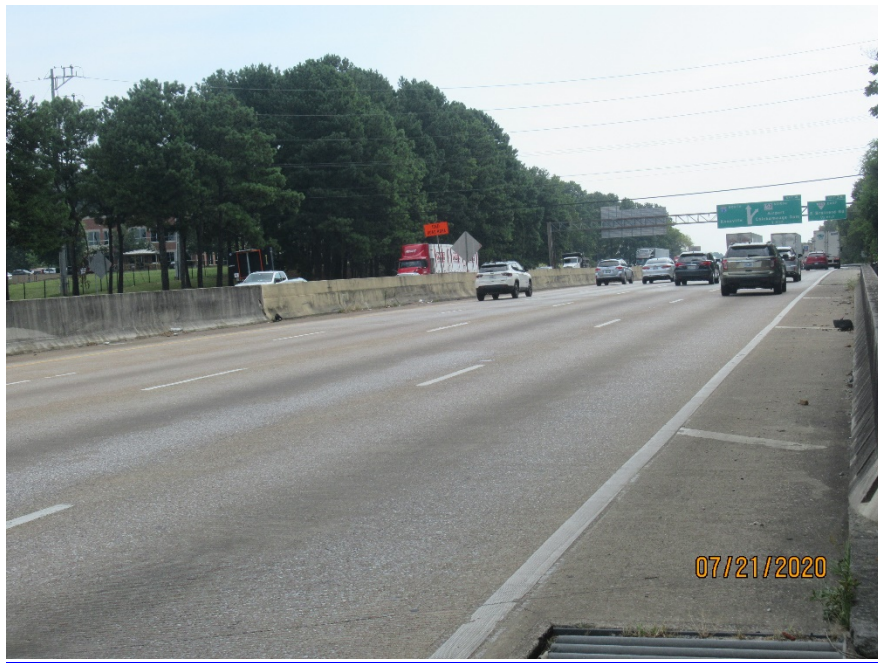
LOOKING ACROSS TOP OF DECK - AHEAD
