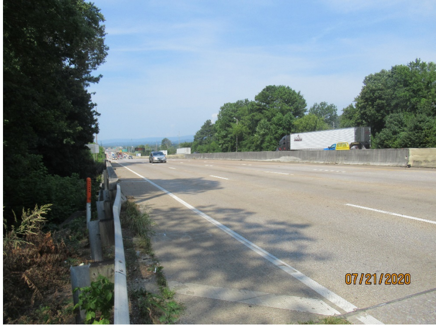
LOOKING BACK ON STRUCTURE - RT, NORTHBOUND
