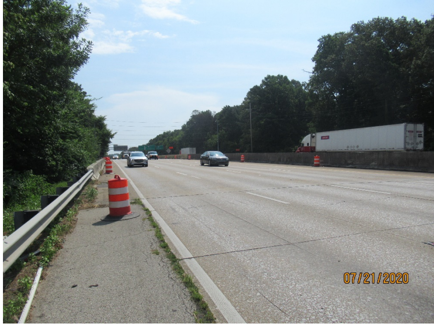
LOOKING AHEAD ON STRUCTURE - LT, SOUTHBOUND
